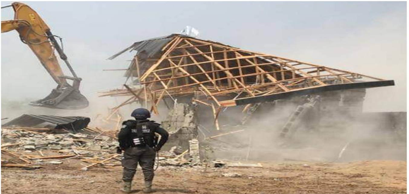
Security protection for demolition of a house in Lagos
